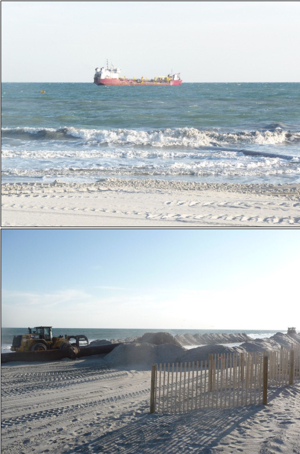
Figure III-63. Hopper Dredge Operation (Bogue Banks)
